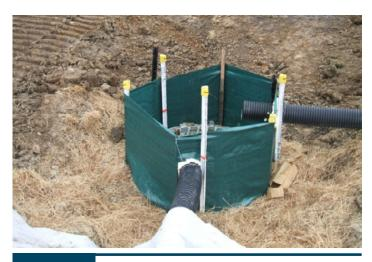
Good use of a silt fence installed to protect a new stormwater catchpit where impounded water will not create a flooding hazard
