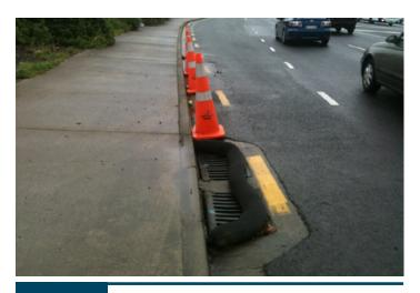
Installation of a silt sock to provide some protection to the catchpit
